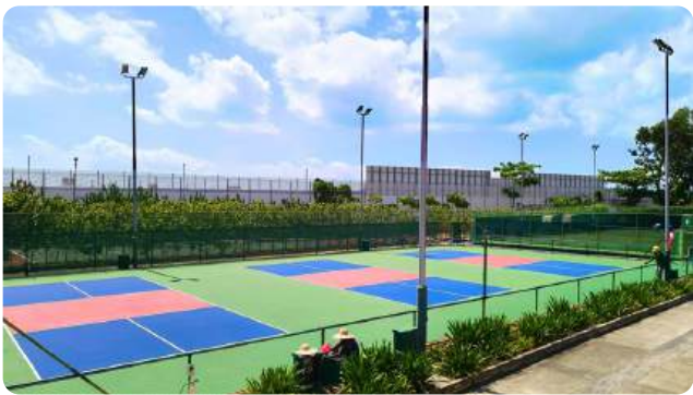
Tennis Court #4 is being converted into three competition-grade pickleball courts to support Members' growing pursuit of the sport, slated for completion in Q1 FY2026.
