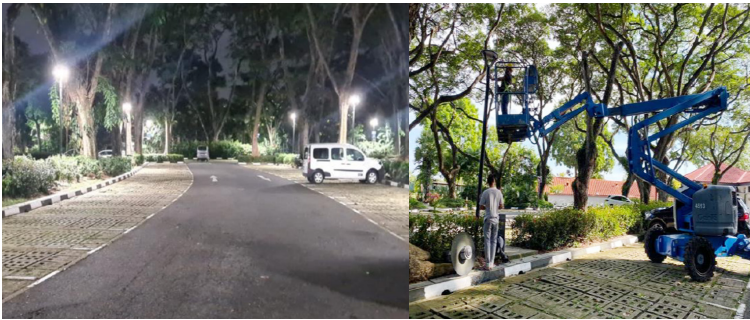
Installation of 52 new LED lights that illuminate the Garden Course Carpark.
