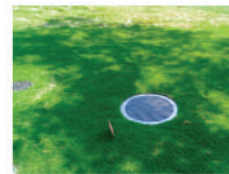
11. New sump added to facilitate better drainage
