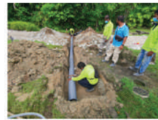
8. Creating subsoil pipe across the buggy path
