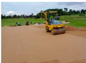
18. Compacting before re-turfing
