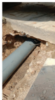
14. 200mm solid pipe that runs below the buggy path
