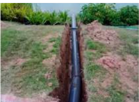
17. New 250mm diameter outlet pipe to drain off water to the lake
