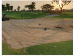
15. Final shaping before turfing
