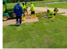
19. Re-turfing back with harvested turf
