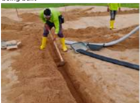
13. Manually trenching to lay mega flow sub soil pipe
