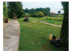
12. Returfing once casting of new buggy path is done
