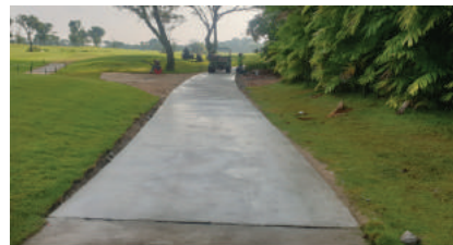
18. New buggy path at the finished level. No signs of ponding after a heavy downpour
