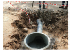
9. New sump with drainage added
