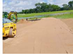
6. Compacting the sand further
