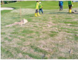
16. Re-turf and topdress with sand
