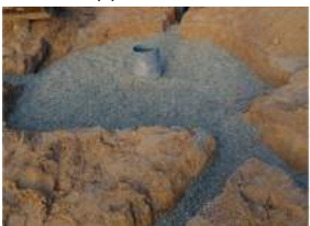
16. Mega flow join to the newly created sump
