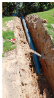
15. 200mm solid pipe that joins straight from the sump to the lake
