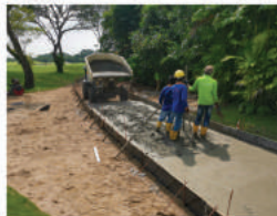
5. Pouring of cement onsite
