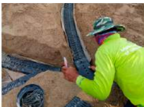
14. Connecting mega flow sub soil pipe
