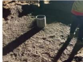
12. Gravel around the sump for better drainage
