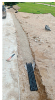
16. Mega flow subsoil along the buggy path
