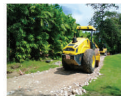
3. Crushed and compacted with a roller
