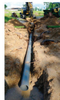
13. 200mm solid pipe join from sump
