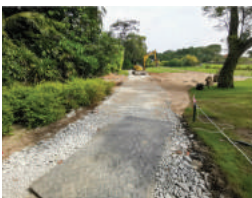
1. Existing buggy path was hacked out
