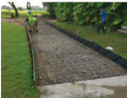
4. Foam works, and reinforcement bar added
