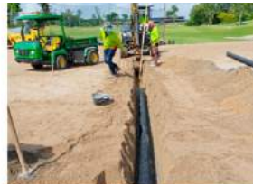
9. 150mm diameter sub soil pipe
