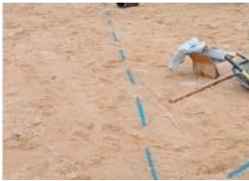
7. Marking out sub soil drainage
