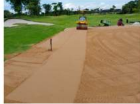
5. Shaped to tie in with existing gradient
