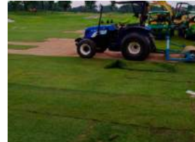
20. Re-turfing with roll turf from contractor's nursery
