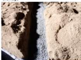
15. Gravel added onto the mega flow pipe
