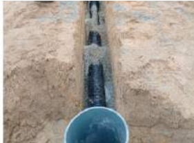
11. Connecting the sub soil pipe to the sump
