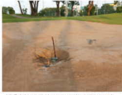
14. Existing sprinklers were raised up to match the new level.
