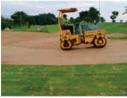
13. Roll to compact and smoothen the surface
