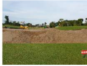
3. Backfill of fresh sand. (Approx. 600-800mm)
