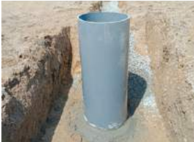
10. New 300mm diameter sump is being built
