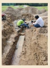
3. Installing new sub soil pipe
