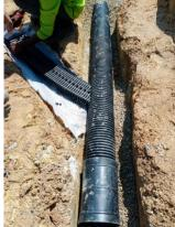
2. Joining the mega flow with a 150mm dia round pipe
