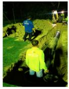
2. 450mm dia sub soil pipe towards the canal.
