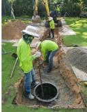
3. Backfill with gravel then with sand.
