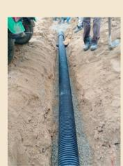
5. New sub soil pipe joined to a new sump
