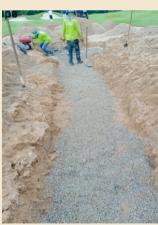
8. Sub soil pipe backfill with new gravel
