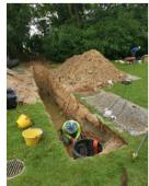
1. 900mm dia catch basin. Existing area ponding with water
